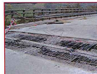
Old joint demolition
