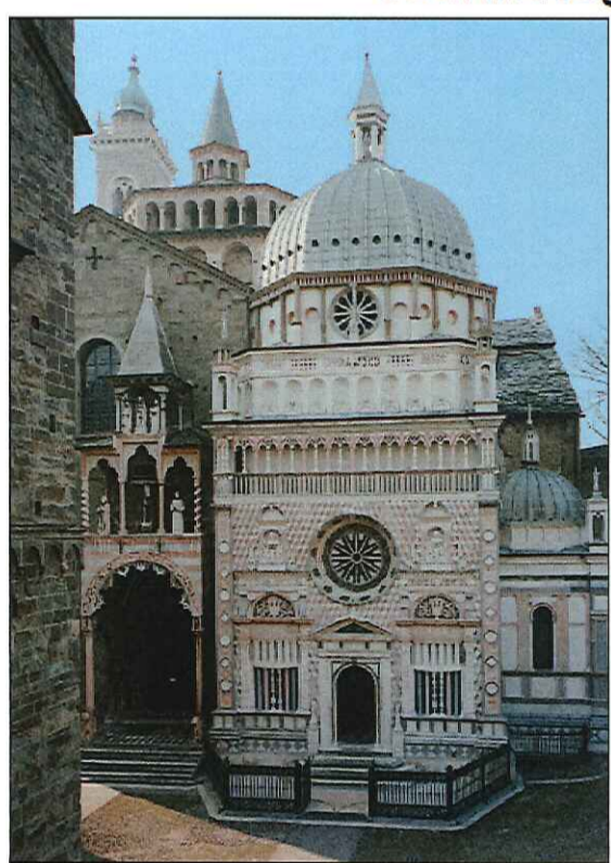
Colleoni Chapel - Bergamo Prestigious monument of Italian Renaissance erected in XV th century. Restoration on 19 marbles & stones started on 1988 and completed on 1990. Presently (2013): 23 years after restoration perfect conservation and durability of SPART® Products & Technologies
